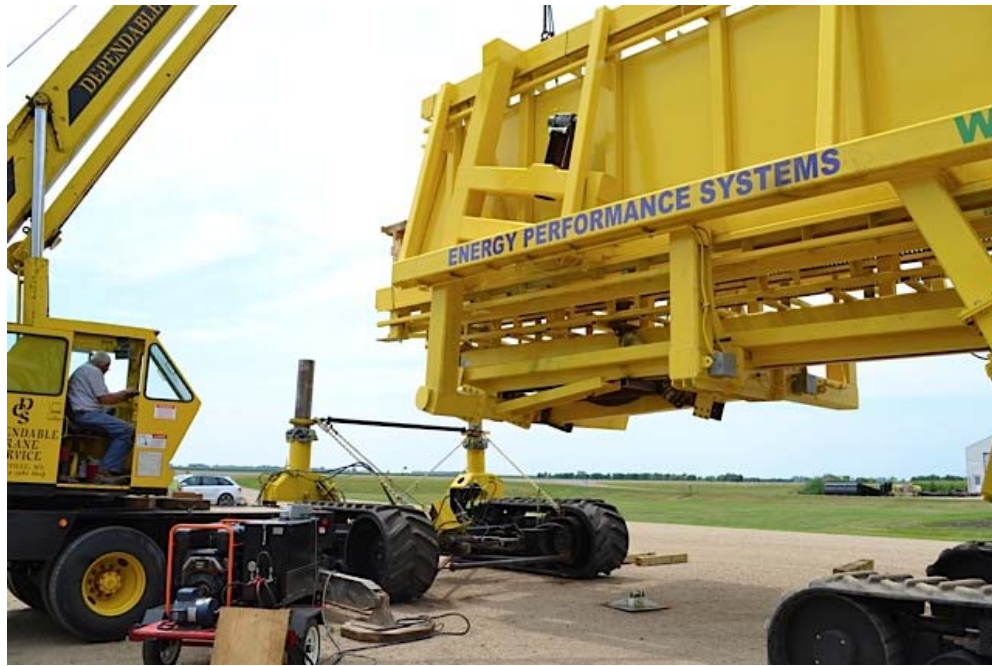
Figure 4. Installing Front Tracks During Field Assembly
